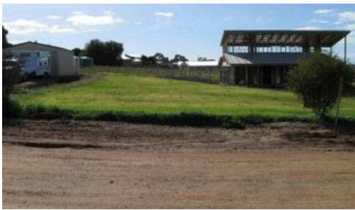
Lot 9 Ardrossan Road, Maitland
