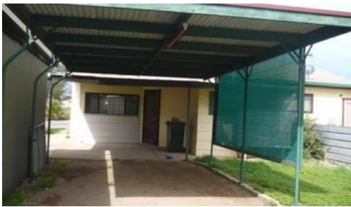
16 Revell Street, Port Pirie
