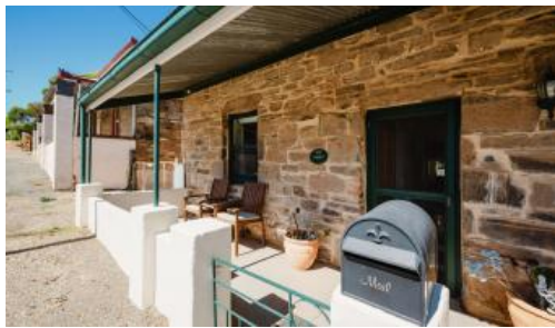
6 Bridge Street East, Burra
