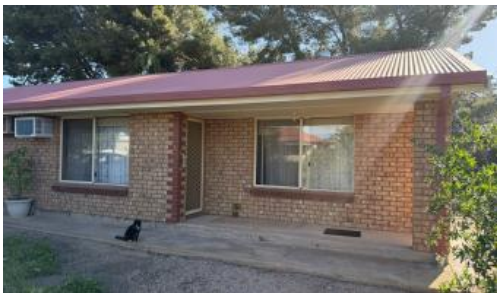
Unit 1, 30 Elizabeth Street, Port Pirie
