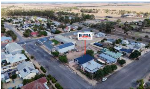
28 Caroline Street, Maitland
