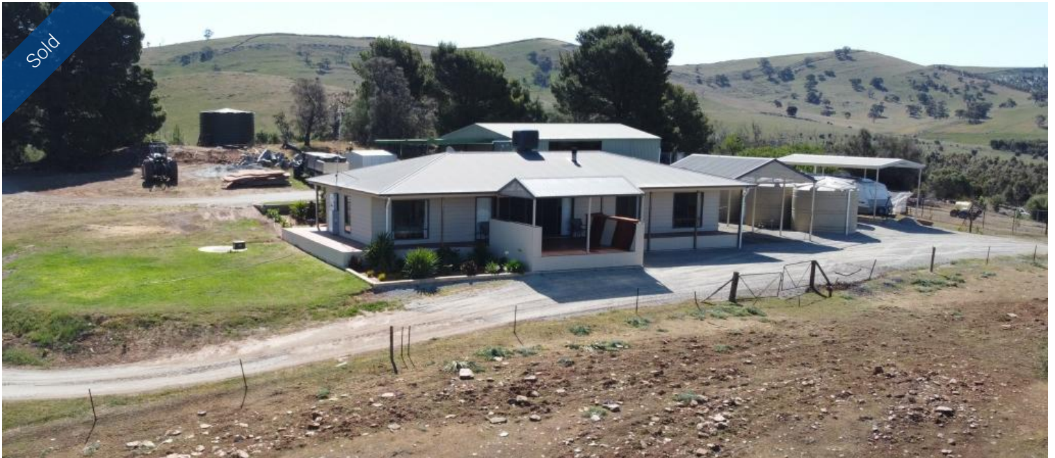
78 Wehrmann Road, Bundaleer Gardens
